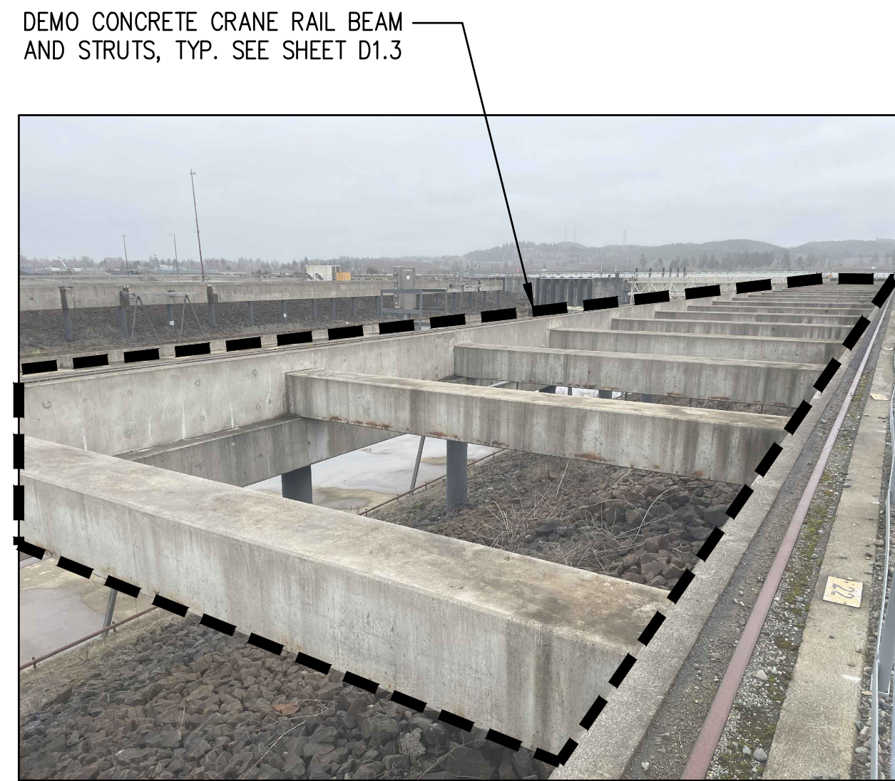
P4 PHOTO DEMOLISH CRANE RAIL SYSTEM, TYP
