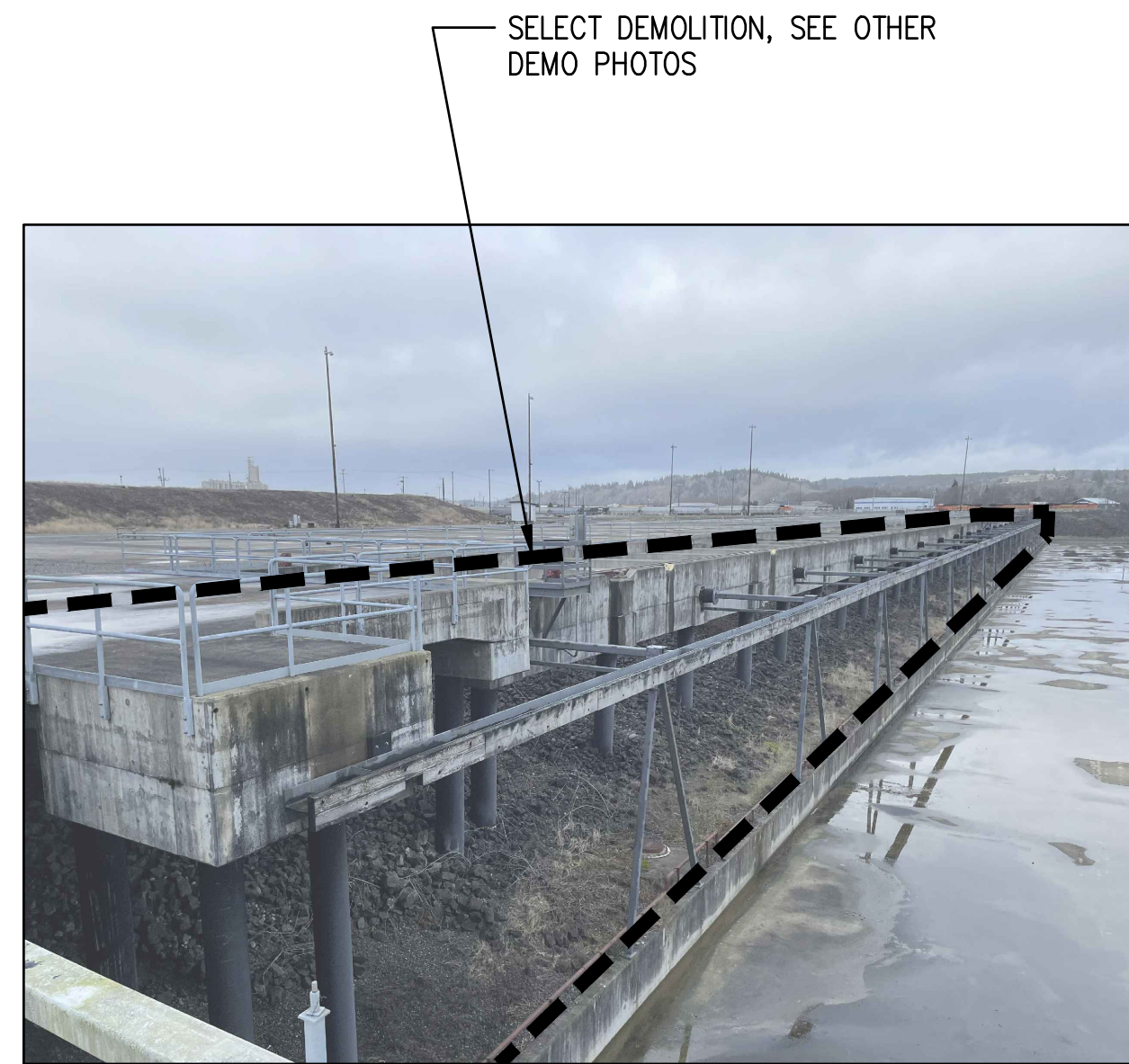
P1 PHOTO DEMOLISH WEST CRANE RAIL AND FENDER SYSTEM
