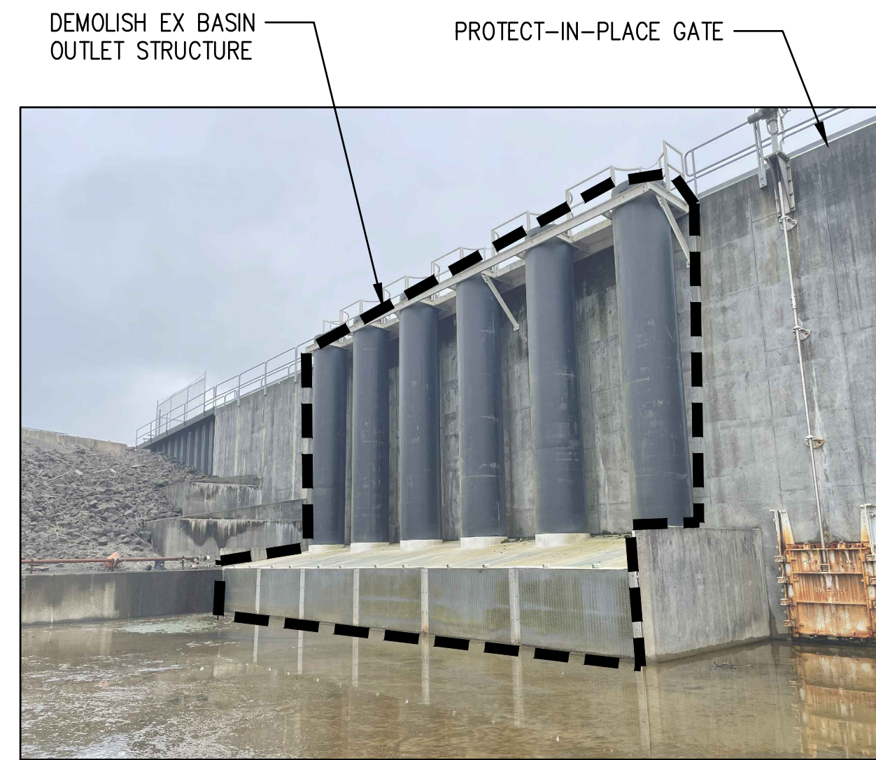
P5 PHOTO DEMOLISH BASIN OUTLET STRUCTURE
