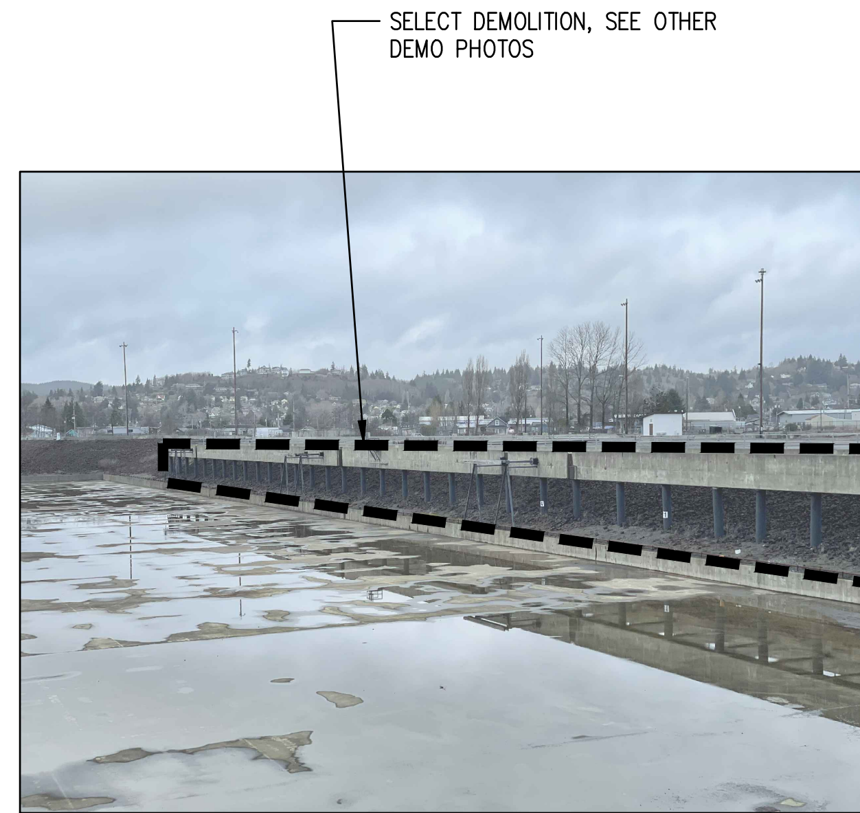
P2 PHOTO DEMOLISH EAST CRANE RAIL AND FENDER SYSTEM
